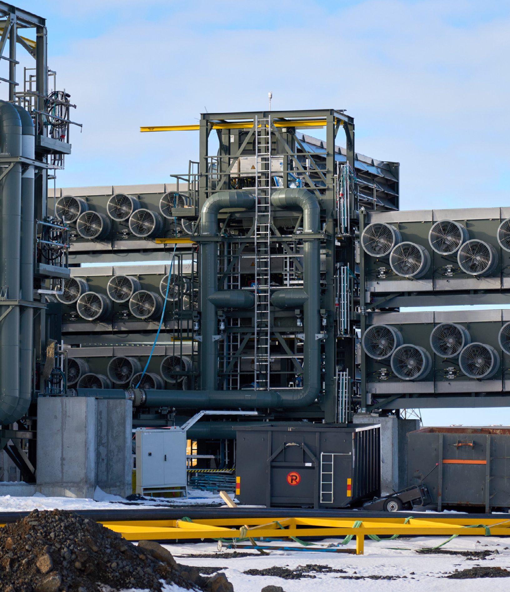
Carbon capture and sequestration machine under construction © Adam Sébire/Stocksy
